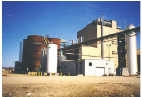
Completed refinery, pumphouse, clay silo, nitrogen generator, tank farm and pipe bridge to loadout
