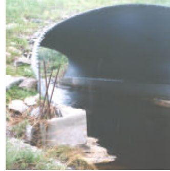
Deacon Creek Arch Pipe
